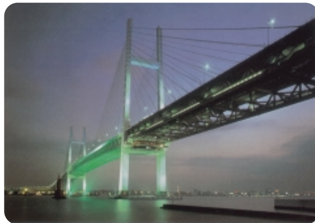
Yokohama Bay Bridge
